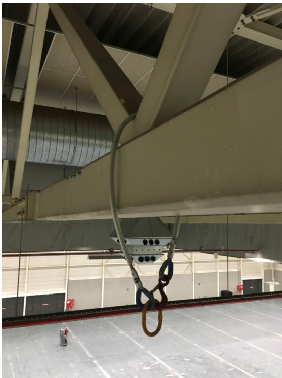
Figure 13: Attachment in truss joint on the lower beam (●)
