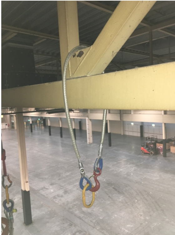
Figure 4: Attachment in truss joint on the lower beam (●)
