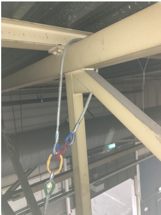
Figure 5: Attachment in truss joint on the upper beam (●)
