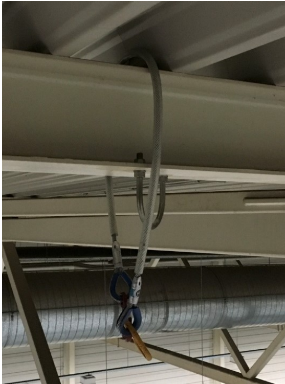
Figure 12: Attachment at girder's suspension points (●)
