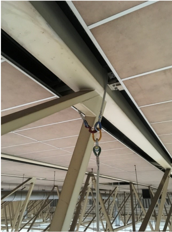
Figure 8: Attachment in truss joint on the upper beam ( ● )
