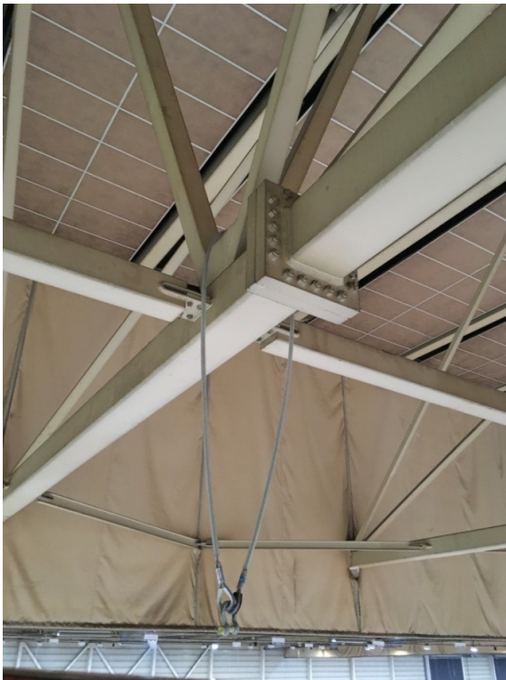
Figure 9: Attachment in truss joint on the lower beam ( ● )
